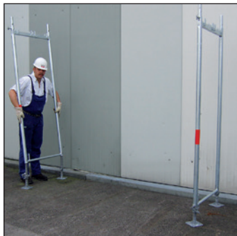
Assemble vertical frame
