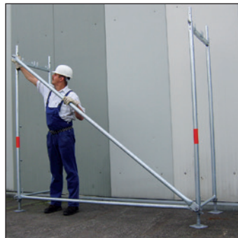
Assemble vertical brace
