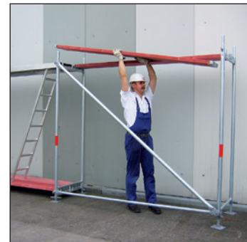
Assemble decks from lower level
