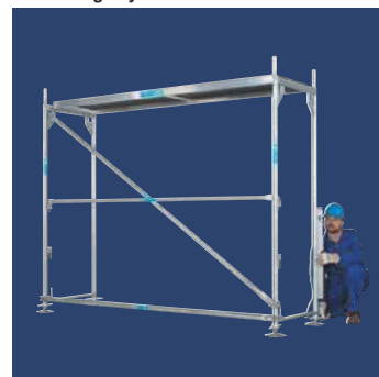
Fit horizontal ledger and level out scaffolding bay
