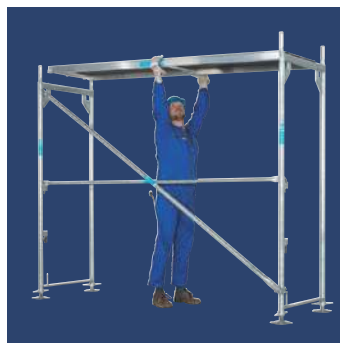
Add vertical brace and deck
