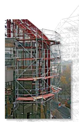
Sufficient work experience of Plettac fitters allows to erect suspension constructions (from top to underside) providing installation of working platforms on any height of building.
